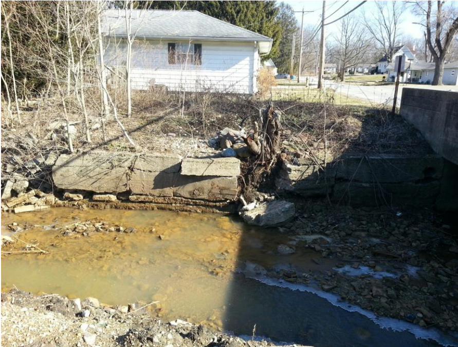
Look East at retaining wall failure near the north east corner of Keegan Street bridge over Grape Creek
