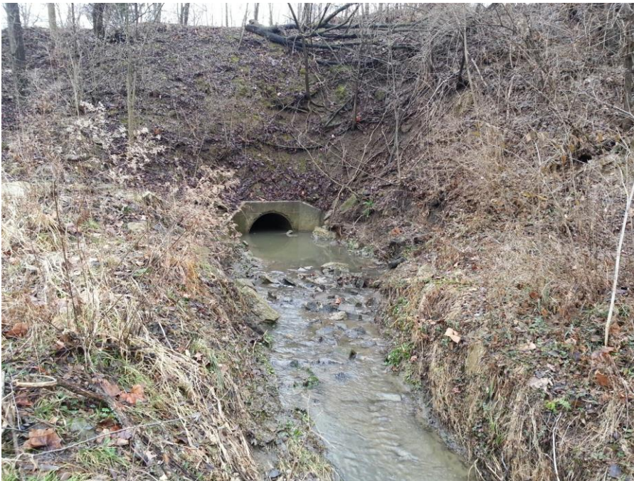
Look at 42 inch concrete discharge at the northeast corner of East 1st Street
