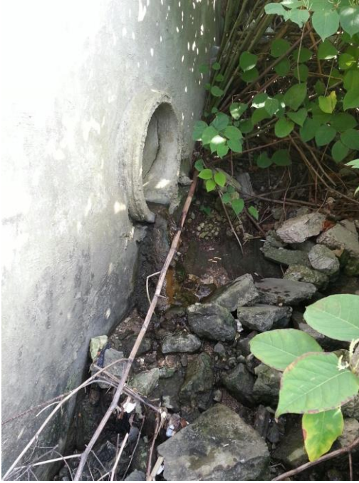
Look southeasterly at Southwest corner of triple barrel box culvert at Route 1 and Grape Creek. Sample Location 16. This is discharge from IDOT storm sewer.
