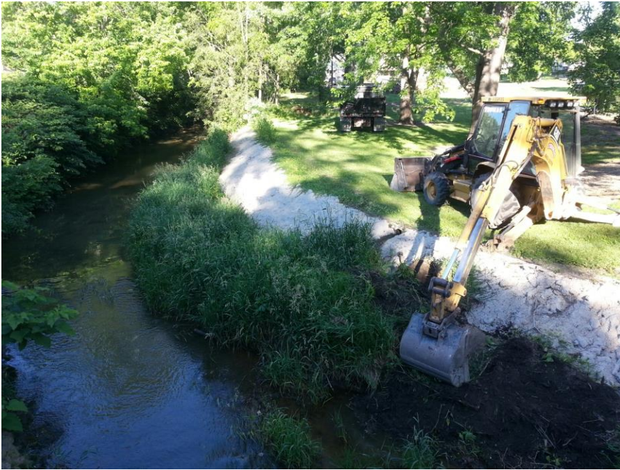
Look westerly at backhoe operator removing sediment build upstream of Washington Avenue Bridge along Grape Creek north concrete bank
