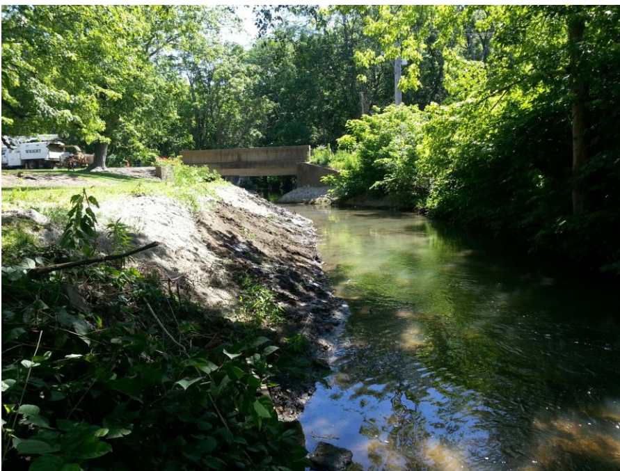
Look easterly along Grape Creek Upstream of Washington Avenue Bridge where 25 cubic yards sediment removed along northern concrete bank
