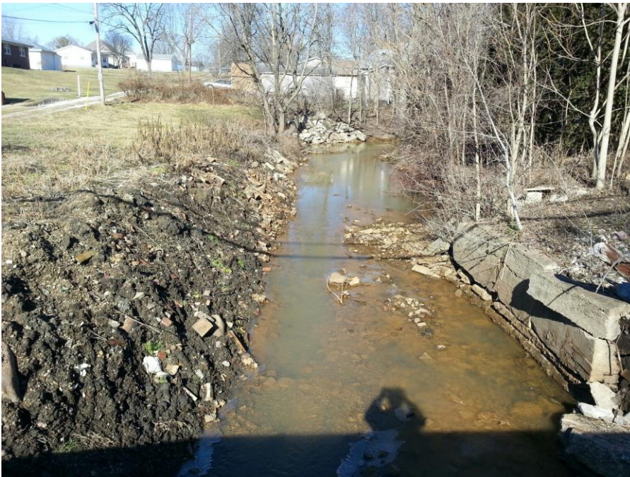
Look northerly from Keegan Street Bridge toward Downstream of Grape Creek where Bank debris build-up was previously removed and riprap placed on Bend. Establish turf and/or erosion control on along west bank.
