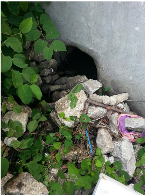
Look northeasterly at discharge at northwest corner of IL Rt 1 and Grape Creek Triple barrel box culvert. Sample Location 17. This is IDOT storm sewer. Regularly remove trash and debris. Consider removing a few pieces of stones to allow full capacity flow of discharge.
