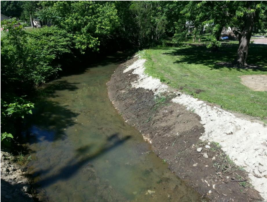
Look westerly from Washington Avenue Bridge over Grape Creek after 25 cubic yards sediment removed from northern bank
