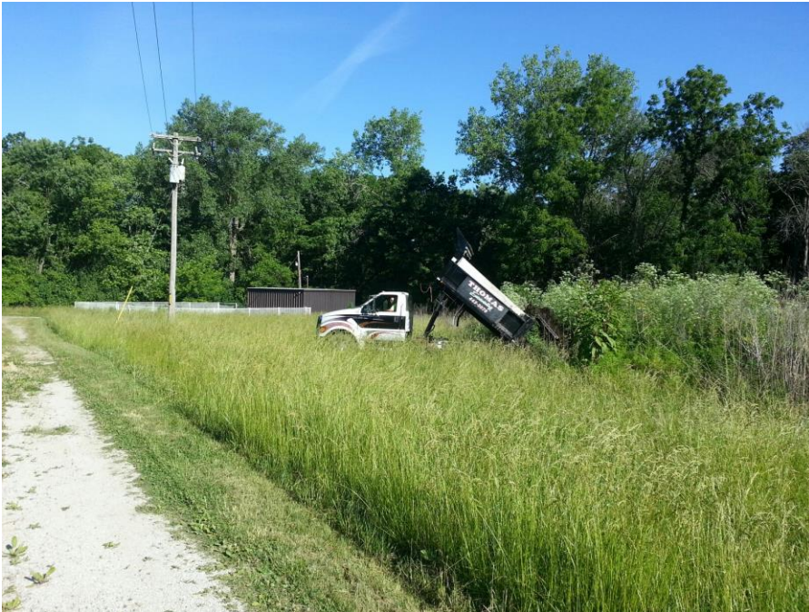
Look westerly at ton truck dumping sediment on top of bank at deactivated Sludge Lagoon void from previous sewage treatment plant now reported to Tilton
