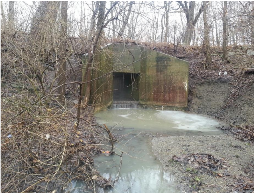
Look southerly at concrete box Culvert Downstream side under Songer Cemetery Road. Ice on ponding water at downstream side
