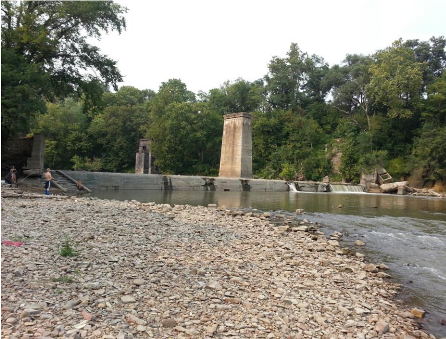
Look from the downstream side of Vermilion River Dam at water pouring over crevice in Dam during low-flow season instead of through the fish ladder
