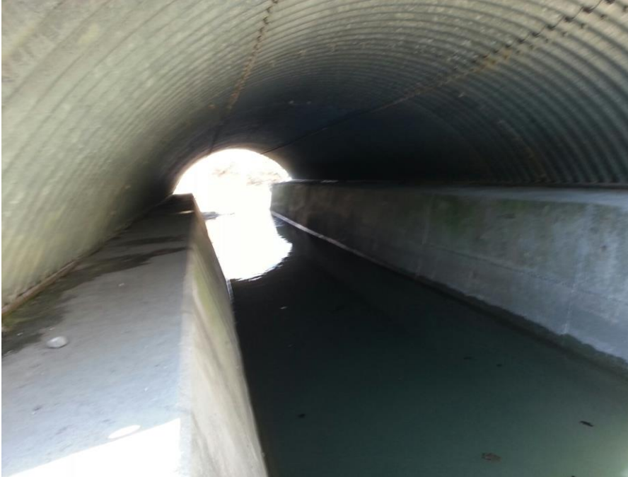
Look from upstream side of corrugated metal culvert at the West Culvert under Norfolk Southern Railroad north of west end of West Ross Lane at Grape Creek
