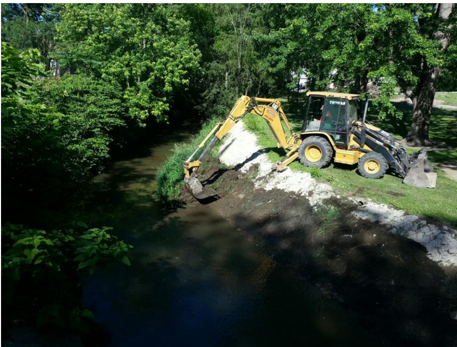
Look easterly at backhoe removing sediment obstructing Tilton drainage along Grape Creek upstream of Washington Avenue Bridge
